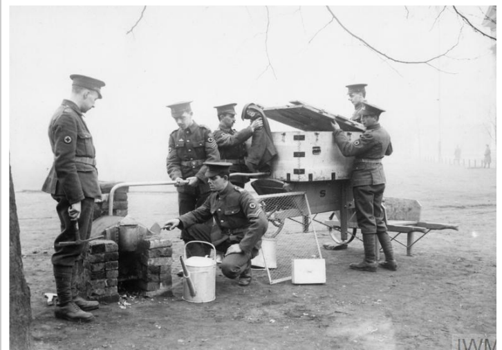
FIG. 1.—PORTABLE STEAM DISINFECTING APPARATUS (THE THRESH)
